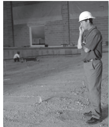
District architect, David Kaye, checks on the progress of the new auditorium at Burger Middle School.
